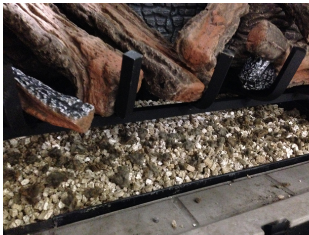
Figure 21 - Completed Installation of Vermiculite and Embers
