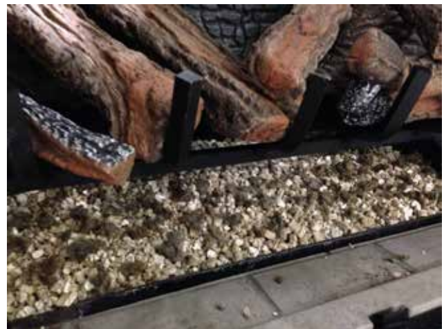
Figure 22 - Completed Installation of Vermiculite and Embers
