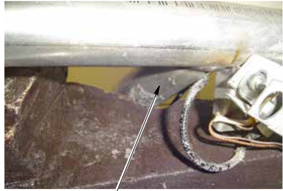
Vertical Portion of Burner Tube
