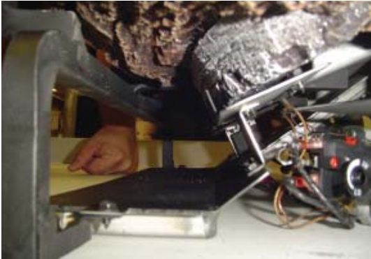
Figure 22C - Installing Right Front Log, Side View
