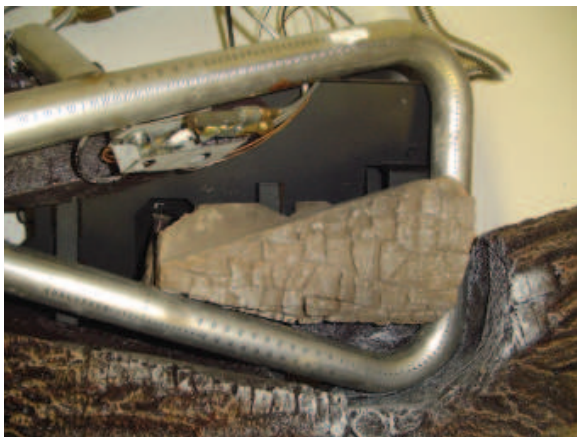
Figure 27A - Installing Charred Log Top View
