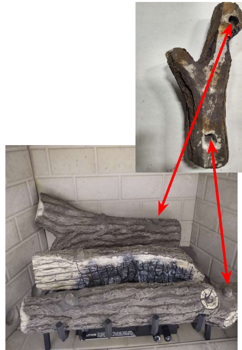
Figure G - Top Right Log Placement
