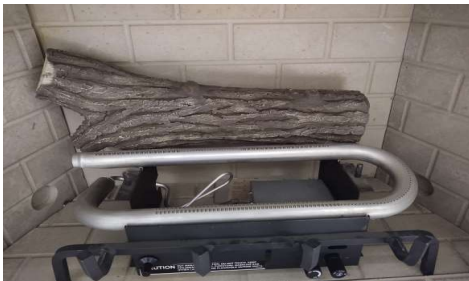
Figure B - Install Rear Log
