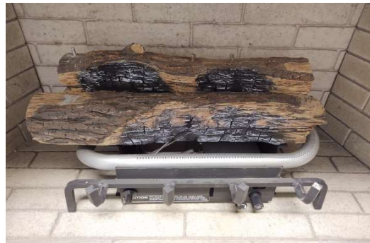
Figure R - Install Middle Log
