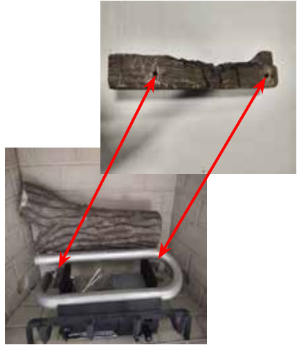
Figure C - Middle Log Placement
