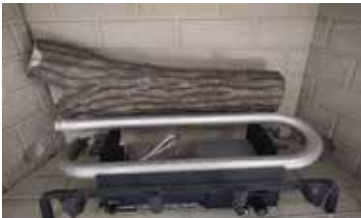
Figure B - Install Rear Log
