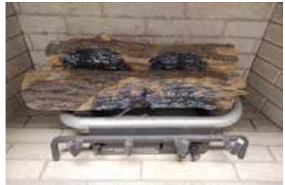
Figure R - Install Middle Log
