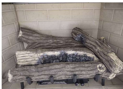
Figure H - Install Right Top Log
