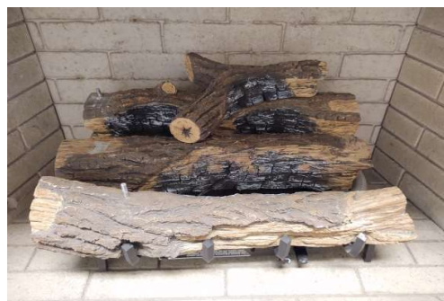
Figure V - Install Top Middle Log
