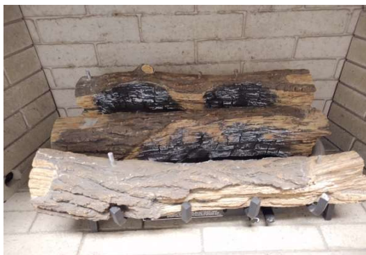
Figure T - Install Front Log
