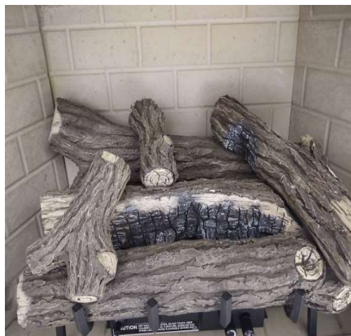
Figure M - Install Top Middle Log
