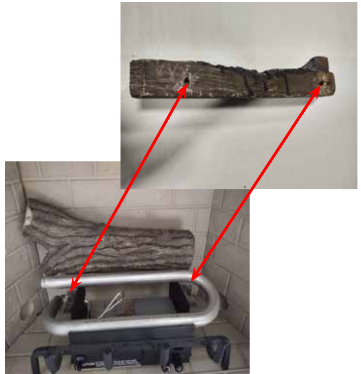
Figure C - Middle Log Placement
