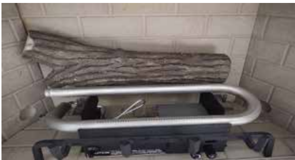
Figure B - Install Rear Log
