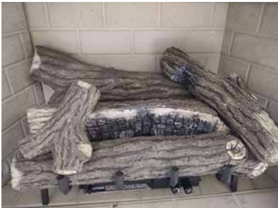
Figure K - Install Top Left Log
