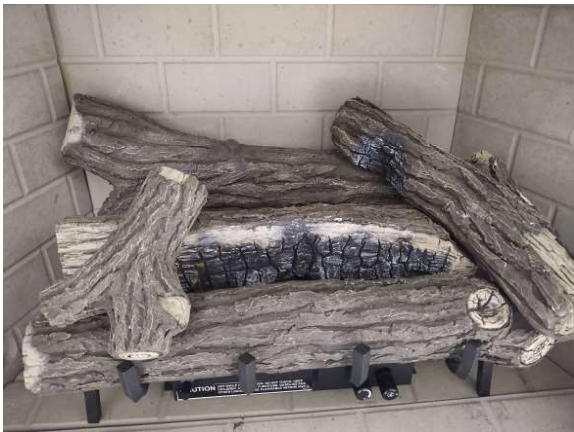
Figure K - Install Top Left Log
