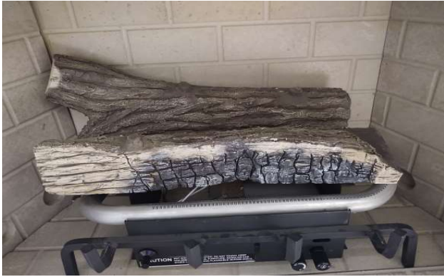
Figure D - Install Middle Log
