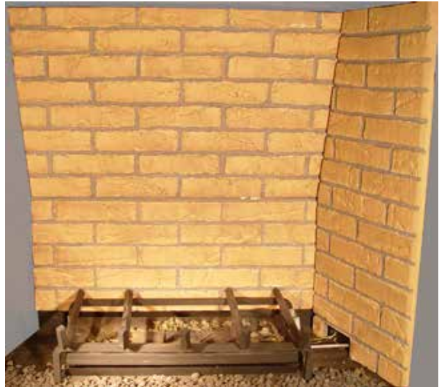
Figure 3: Installing Top, Rear Ceramic Panel
