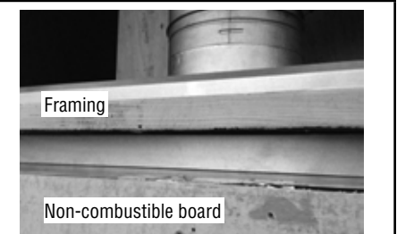
Step 3. Heat shield will now protect framing from heat from flue.
