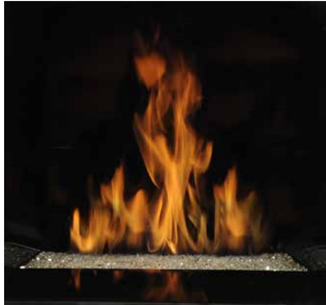
Figure 71—Burner Flame Appearance
