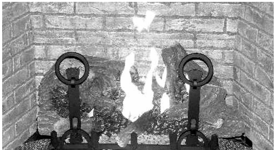
Figure 43 - Burner Flame Appearance
