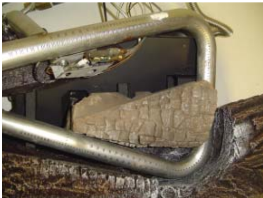
Figure 25A - Installing Charred Log Top View
