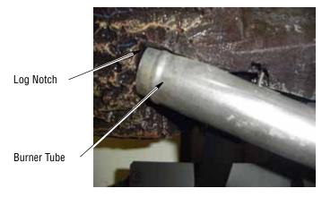
Figure 19A - Installing Back Left Log
