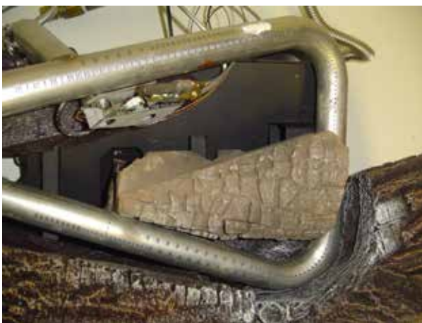
Figure 21A - Installing Charred Log Top View
