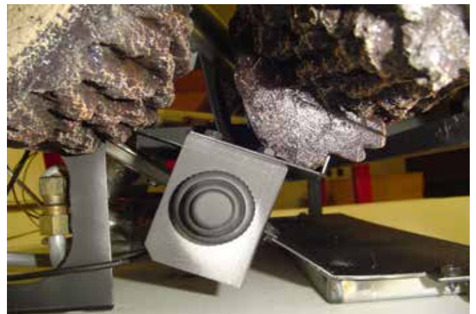
Figure 20A - Installing Front Left Log Side View
