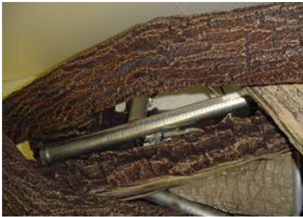
Figure 24A - Installing Back Top Log, Top View
