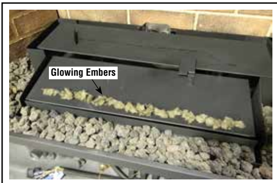
Figure 42 - Install glowing embers
