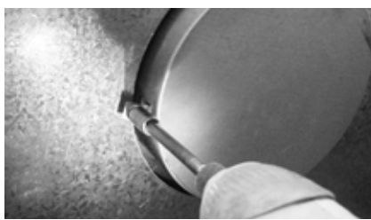
Step 6: Secure the round flue cover (provided) to the wrapper over the rear venting outlet. Use two (2) 3/4" long sheet metal screws
