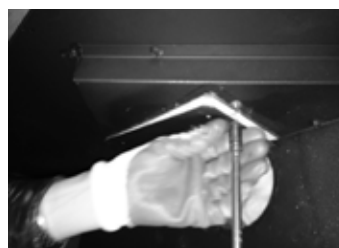
Step 7: Remove the 2 screws holding the block off plate and gasket to top vent flue. Retain screws as they will be re-used.
