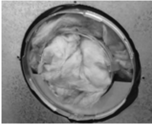
Step 5: Bend tabs out on round flue cover.
