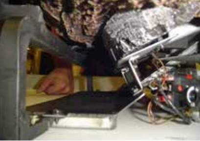
Figure 22C - Installing Right Front Log, Side View
