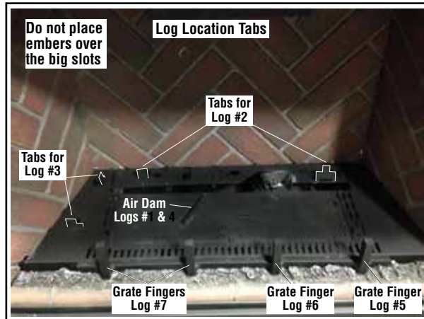
Figure 41 - Locate the log placement tabs
