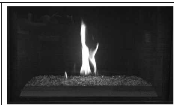
Figure 40 - Contemporary Fireplaces Flame Appearance
