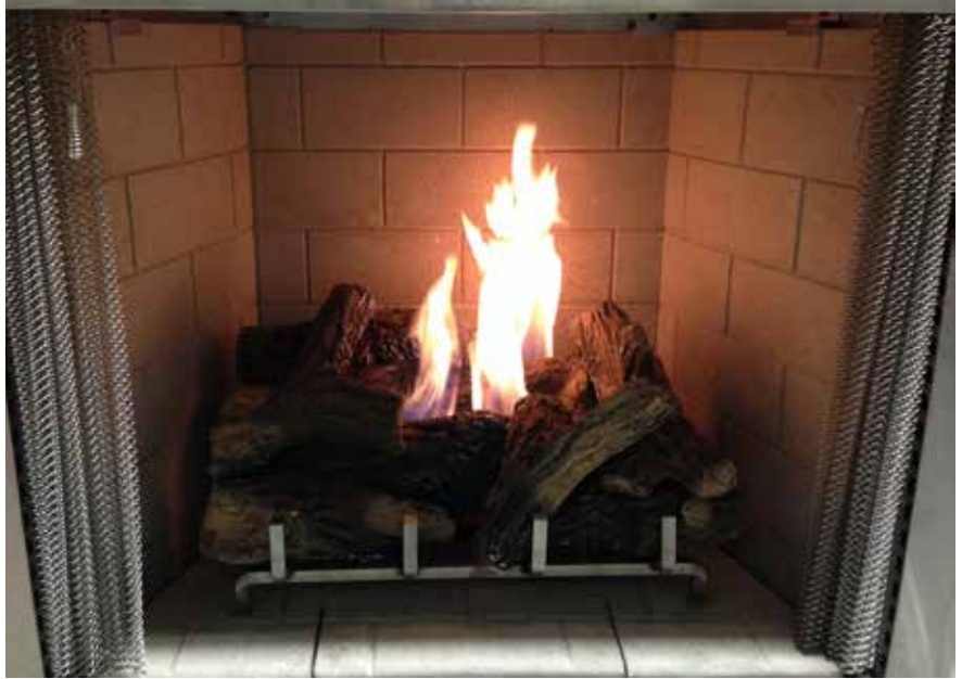
Figure 23 - Proper Burner Flame Appearance
