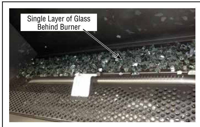
Figure 50 - Placing a Single Layer of Glass Media.
