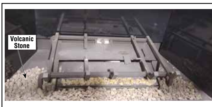
Figure 40 - Install volcanic stone
