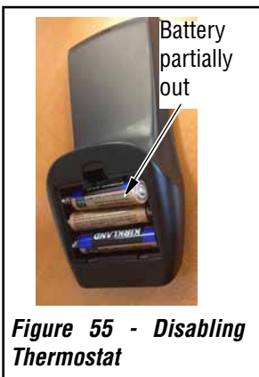
Figure 56 - Disabling Thermostat
