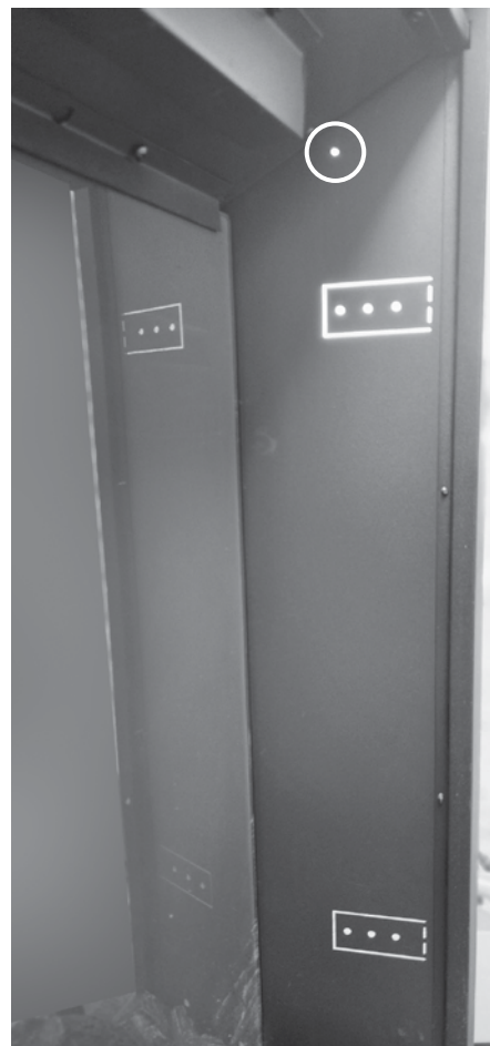
Figure 10 - Secure Fireplace to Framing
