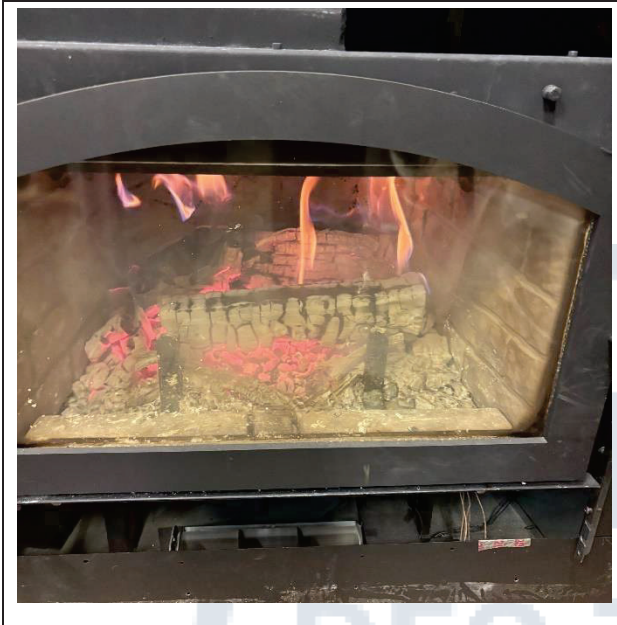
L3 Residual Fuel Loaded
